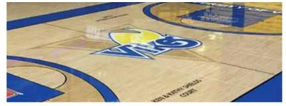
A fixed resilient floor system offering environmental stability combined with high shock absorbing resiliency.
