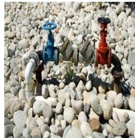
A cross connection is defined as, "Any actual or potential connection between a potable water system and any other source or system through which it is possible to introduce into the public
