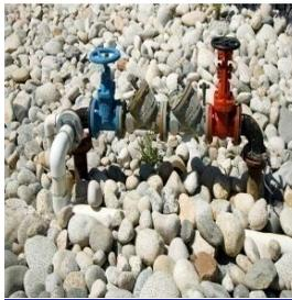
A cross connection is defined as, "Any actual or potential connection between a potable water system and any other source or system through which it is possible to introduce into the public
