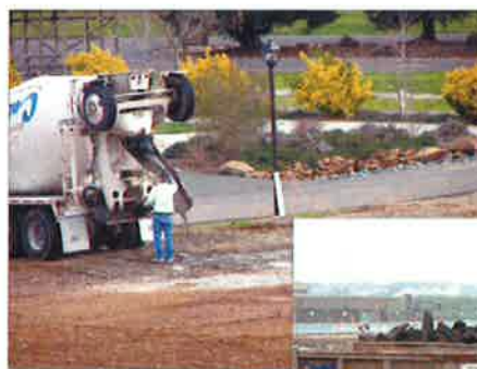
Figure 1. Chute washwater being dumped on the ground
